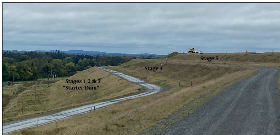
Figure 7: Embankments side profile
